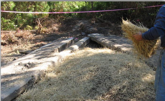
AFTER Reclamation complete of the Dudley airshaft.
